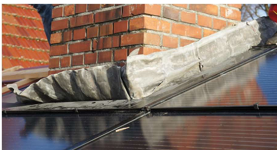
Fig. 3: Joints to chimneys
