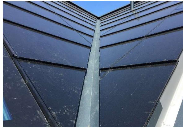
Fig. 2: Formation of a roof valley
