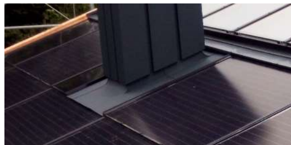
Fig. 4: Dummy modules in area shaded by the chimney
