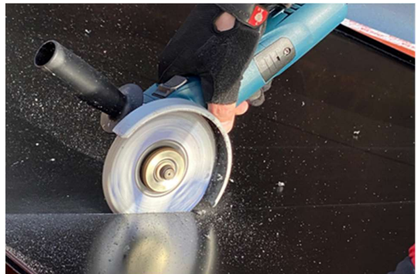
Fig. 11: Cutting with angle grinder
