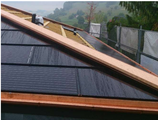
Fig. 1: Finish to the ridge of a hip roof
