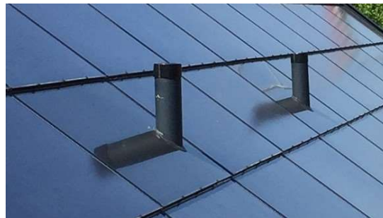
Fig. 6: Dummy modules with opening for ventilation outlets
