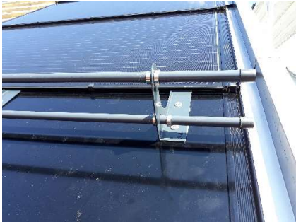
Fig. 5: Eaves area with snow barrier on dummy modules
