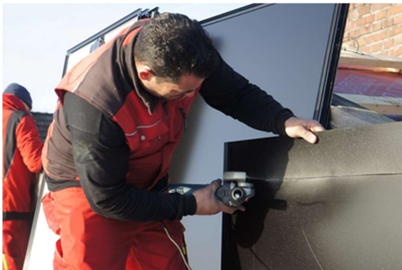
Fig. 10: Cutting dummy module on site
