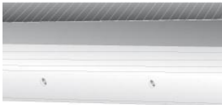
Image 4-24: Holes drilled for potential equalization
