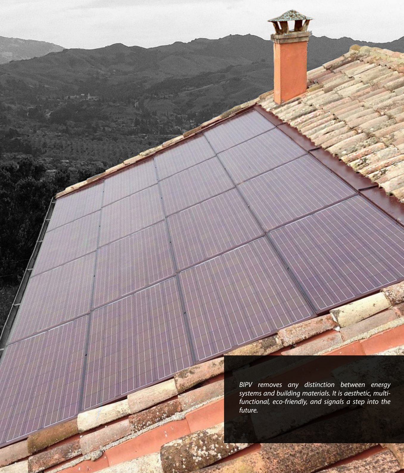
Detail of special BIPV (Solrif®) frame
